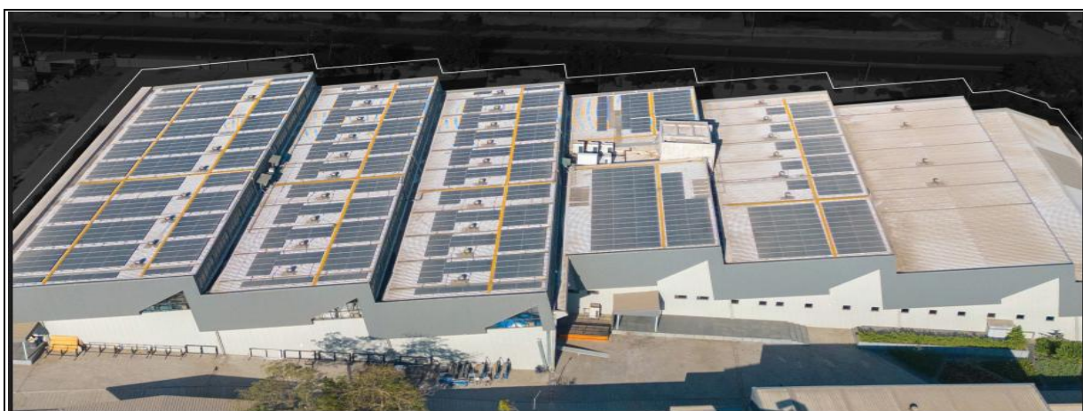
SOLAR PLANT AT MANUFACTURING FACILITY - HRS ALUGLAZE LIMITED
