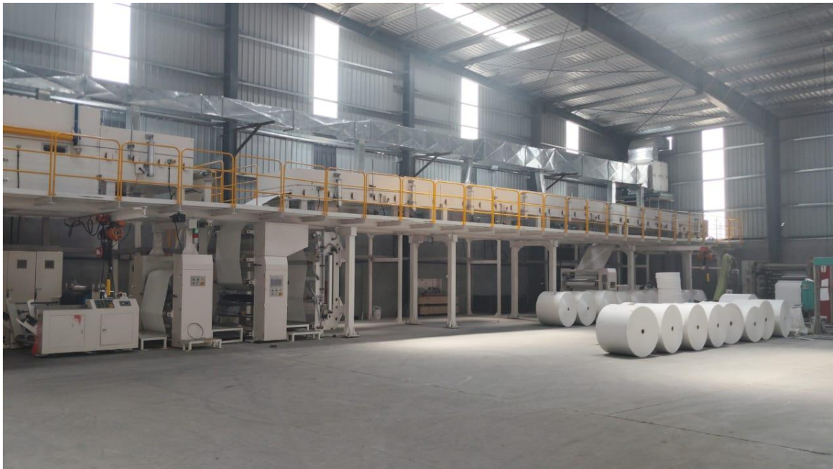
Barrier Coating Machine
