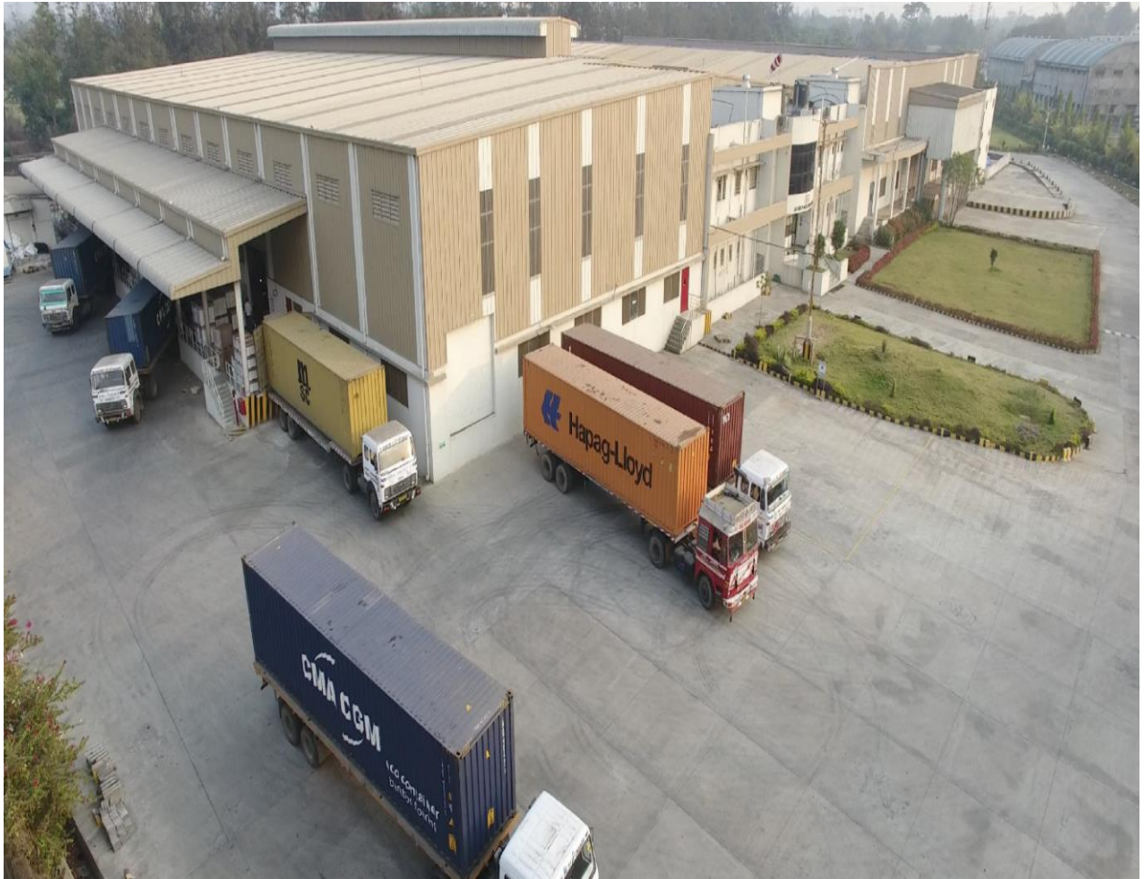
Above: photo of the Silvassa Facility.
